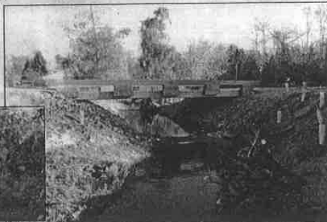
Replacing fish passage barriers, like this culvert, with bridges improves the opportunity for returning salmon to navigate upstream toward Lake Terrell. NSEA replaced this culvert in 2014.
