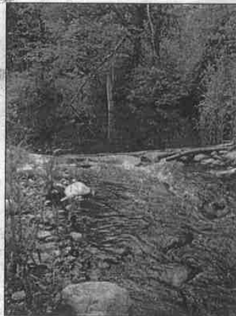
Lake Terrell Dam After
