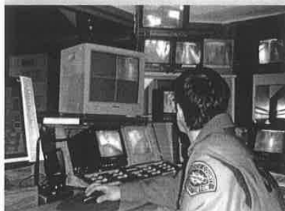
Existing central control room.
