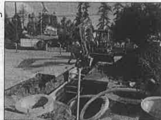
Installing a new culvert under Birch Bay Drive.
