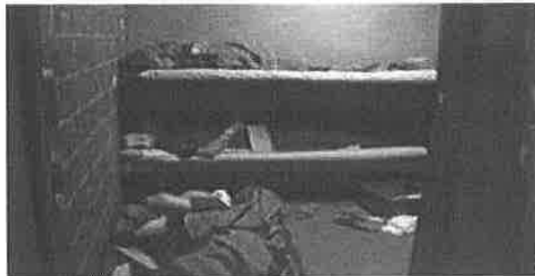
Close Observation cell used for housing offenders with significant and threatening mental health issues is located in the noisy and busy booking area
