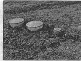
New risers installed on septic tank for easier inspection and maintenance.
