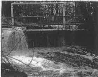
Lake Terrell Dam Before
