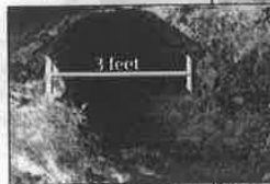
Replacing fish passage barriers, like this culvert, with bridges improves the opportunity for returning salmon to navigate upstream toward Lake Terrell. NSEA replaced this culvert in 2014.
