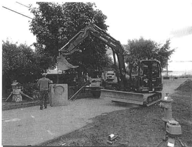
Installing a new stormwater vault on Beachway Drive
